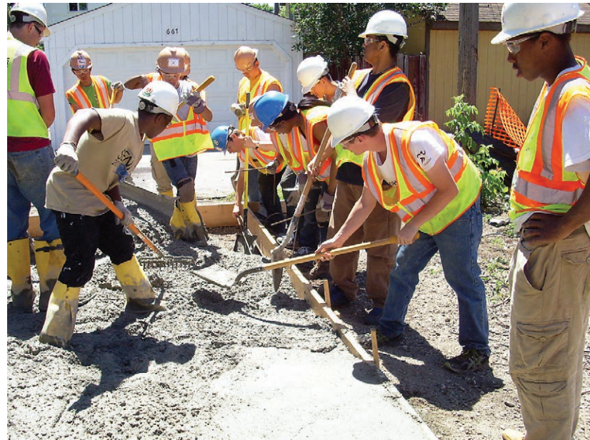
Students working at an UnderConstruction project
